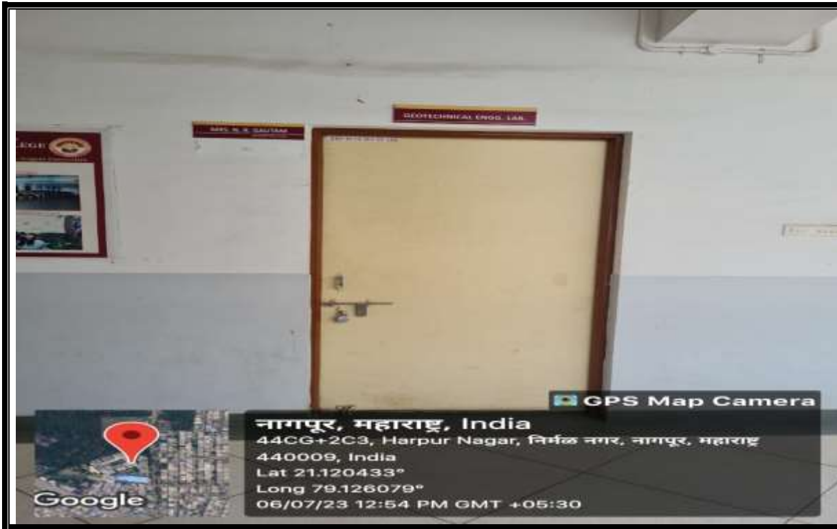
Geotechnical Engineering Lab.(Front View)
