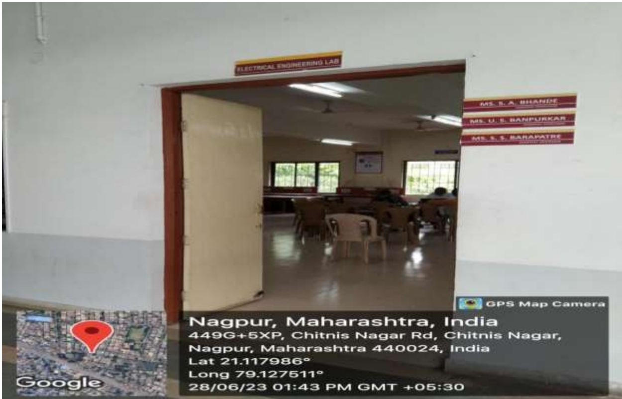
Electrical Engineering (Front View)
